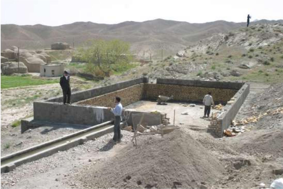
Figure 5 New Water storage being constructed in village of Garmaab Bala. . Courtesy of CENESTA
